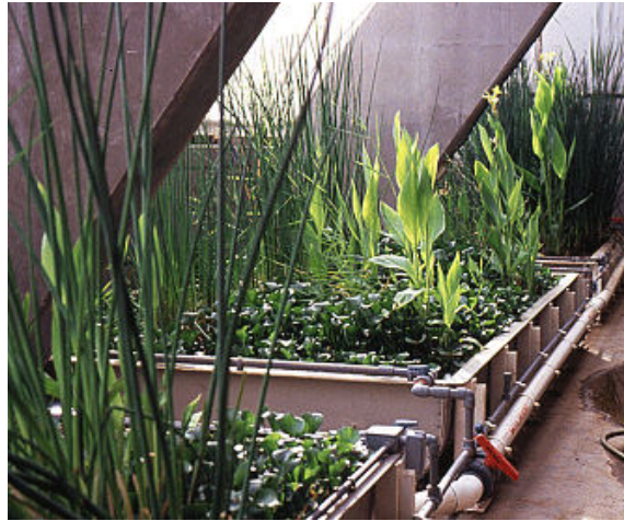
Figure 1. Three of the fiberglass tanks which housed one of the two constructed wetland systems inside Biosphere 2. Shown soon after closure, the system included 14 floating and rooted wetland species and provided additional habitat as well as attractive foliage.
