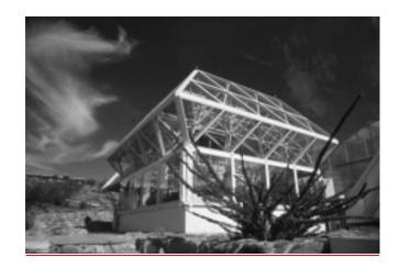
Figure 1. Biosphere 2 Test Module, Oracle, Arizona, a 480 cubic metre volume, glass and spaceframe structure functioned as an experimental facility from 1986-1993.
