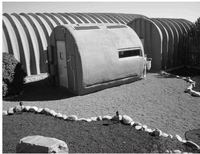
Figure 4. [The Laboratory Biosphere](#), an opaque modular biosphere with side viewing windows, [Santa, Fe, New Mexico](#). The steel cylindrical chamber in front houses the living systems, while the one in the rear contains the variable volume chamber. In the rear, a support workshop and laboratory/computer control rooms.
