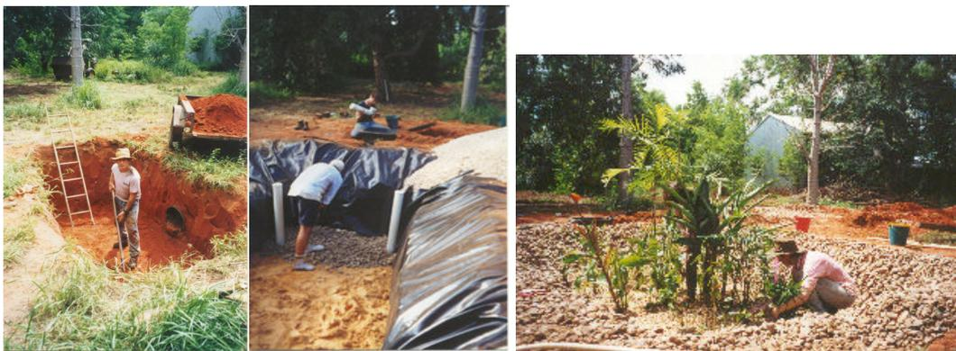
Figure 12. Stages of construction – (left) excavation, (center) installation of pipes and liner, (right) planting of Wastewater Garden, Birdwood Downs homestead, April 2000. Wastewater Gardens can be installed more economically using community labour. Training/education can help people correctly design and install such systems after “hands-on” training.
