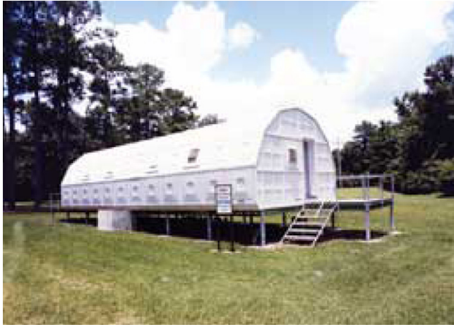
Fig. 1. The Bio-Home at NASA Stennis Center which incorporated indoor constructed wetlands for wastewater treatment and reuse and plant/microbe systems for purifying the indoor air ( http://www.sti.nasa.gov/tto/Spinoff2007/ps_3.html ).
