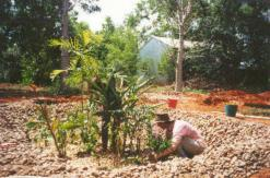
Figure 12. Stages of construction – (left) excavation, (center) installation of pipes and liner, (right) planting of Wastewater Garden, Birdwood Downs homestead, April 2000. Wastewater Gardens can be installed more economically using community labour. Training/education can help people correctly design and install such systems after "hands-on" training.
